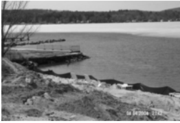
From silt fence and haybales to...
