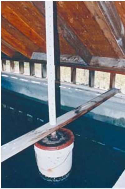
The floating bucket filled with air, and flag pole secured with guide so the wind can't push it over at an angle above the roof. Breezeways are screened.
